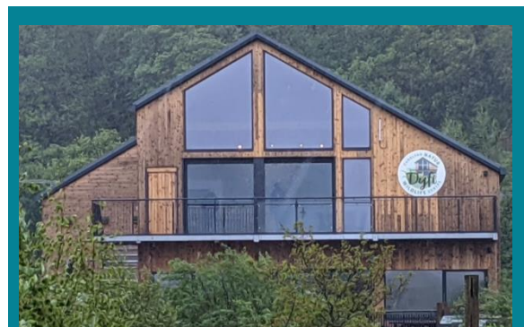
Above and below: Dyfi Wildlife Centre, and solar panels on its roof
